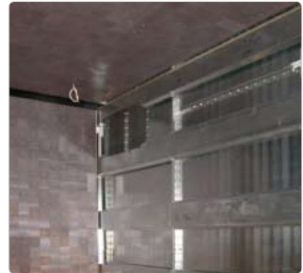
Structure for the installation of ferrite absorbers
